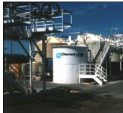
CRS-45 manufacturing and distribution facility.
