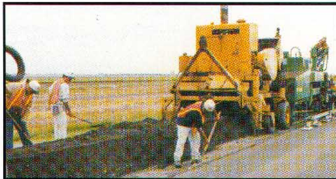
Processed product is put down on the road surface.
